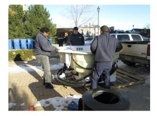
In some cases a crane will be required to lift the hot tub to higher levels of a building. If you must do this be sure the straps are spaced to evenly spread its weight. Also be careful that nothing is touching any of the plumbing or the outside edges of the tub so it will not be damaged during the lift.
