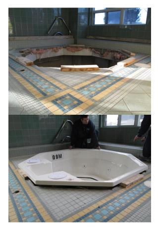
When connecting the plumbing to the hot tub, we recommend using several coils of extra flex pipe under the tub so in the event you need to lift the tub for maintenance you will not have to cut any lines.
